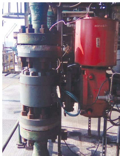
Above: One of several MOGAS 6-inch, ASME 2500 Class C-Series valve sits atop a coke drum in a South American refinery's cutting water application. This industry-proven valve is engineered specifically to perform in high erosion conditions.
