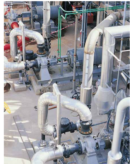
Figure 3. The type HPX single-stage process pump for refinery and petrochemical plant services.
