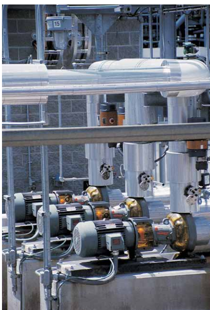
Figure 6. Durco Mark 3 ASME B73.1M standard process pumps for chemical processing applications.
