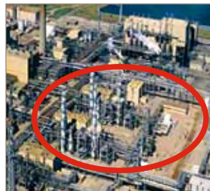
Figure 7 – A Carbon Capture Unit in a Coal-Fired Power Plant (circled area) Source: [1]
