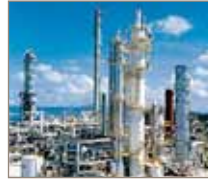
Figure 6 – A Post-Combustion CO 2 Capture Unit Source: [1]
