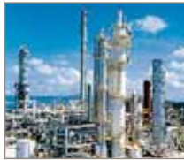
Figure 6 – A Post-Combustion CO 2 Capture Unit Source: [1]
