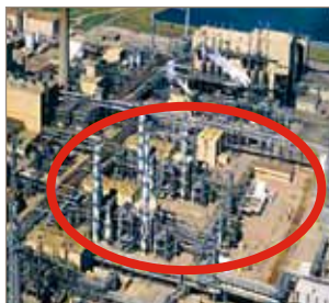
Figure 7 – A Carbon Capture Unit in a Coal-Fired Power Plant (circled area) Source: [1]
